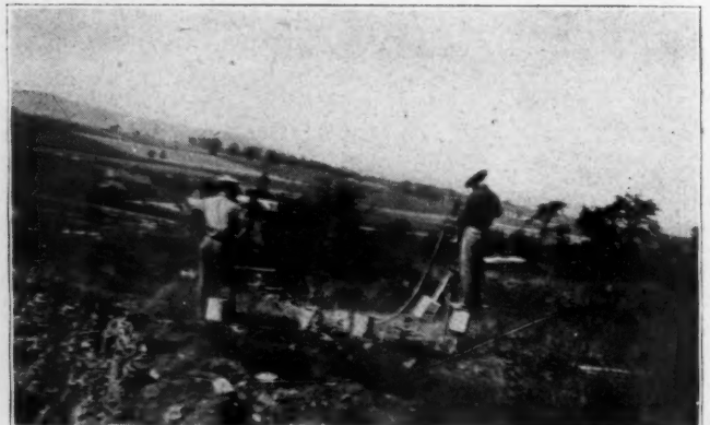
Drilling Crew With Piston Air Drill. Top Number 5 Quarry
